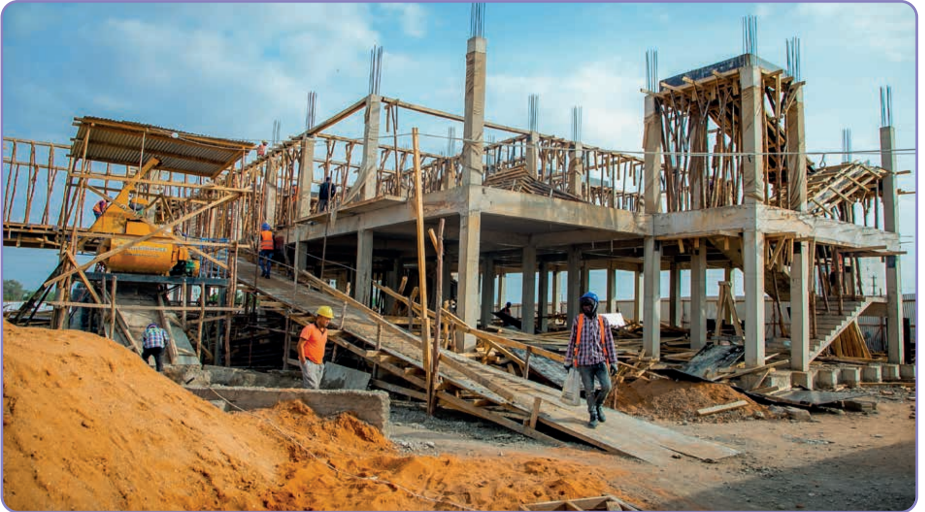
Construction of PPRA Head Office in Dodoma, as captured on December 12, 2022
